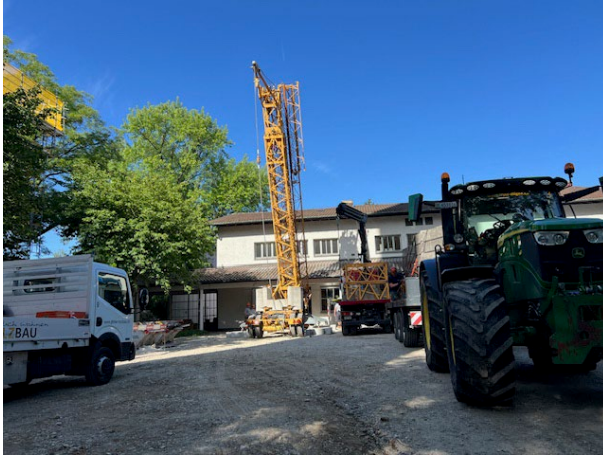
Montage Kran (Fa. Gfeller)
